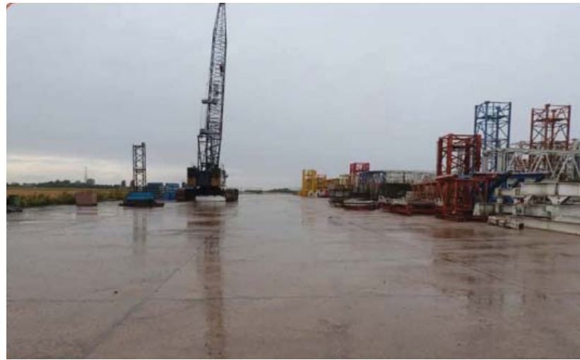
Areas of the site are used for crane equipment storage
